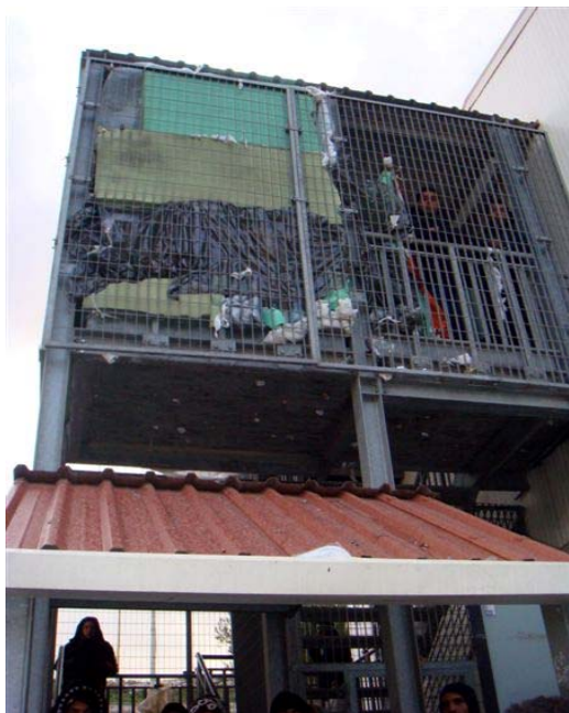
1. Mattresses are placed in the stairwell. external as a "room" due to lack of beds
