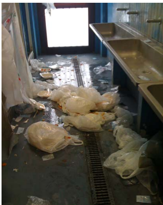
3. Corridor of toilet
