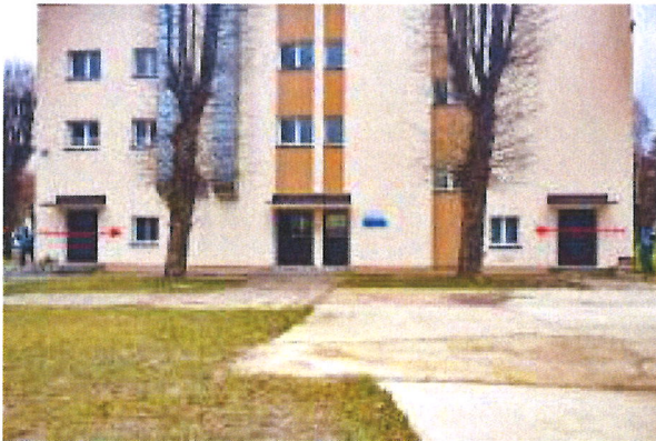
Photo 2.19 Approaching a building from two sides
