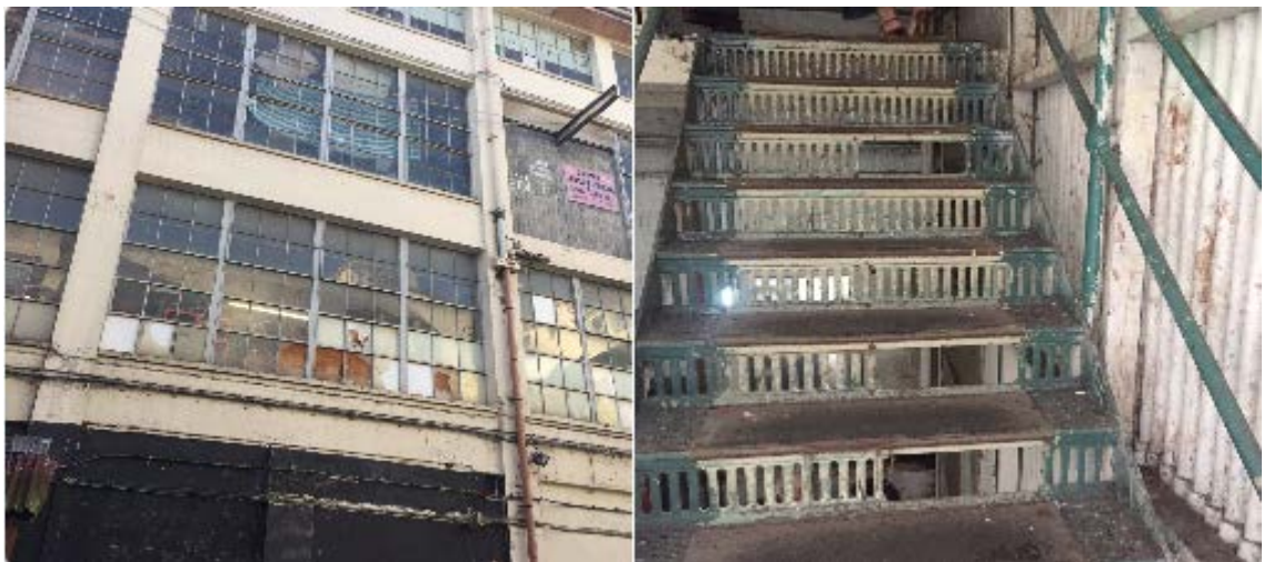
The Leicester Imperial Typewriter Building, where it is estimated that over 50 workplaces are housed. The building is in disrepair and key fire escapes are not fit for purpose.
